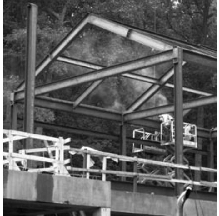
Welders at work on the frame of the center's cafe building.
