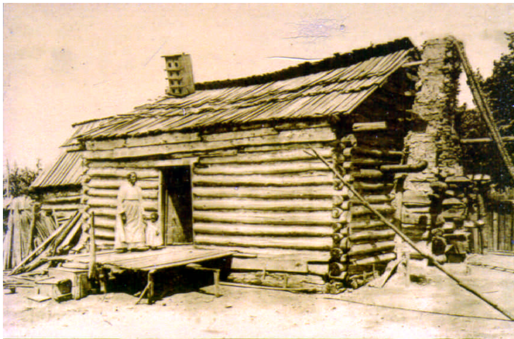
Figure 11. Tidewater example of dwelling employing chimney props.
