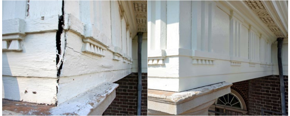
North corner of the entablature before and after restoration. TJF
