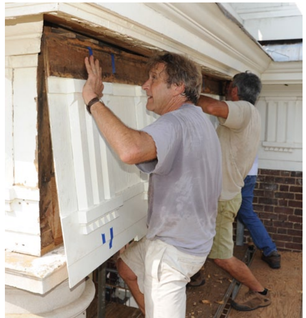
Senior Restoration Specialist Rob Newcomb, Henry Cersley and Bob Self lift the restored entablature back into place. T.J.F.
