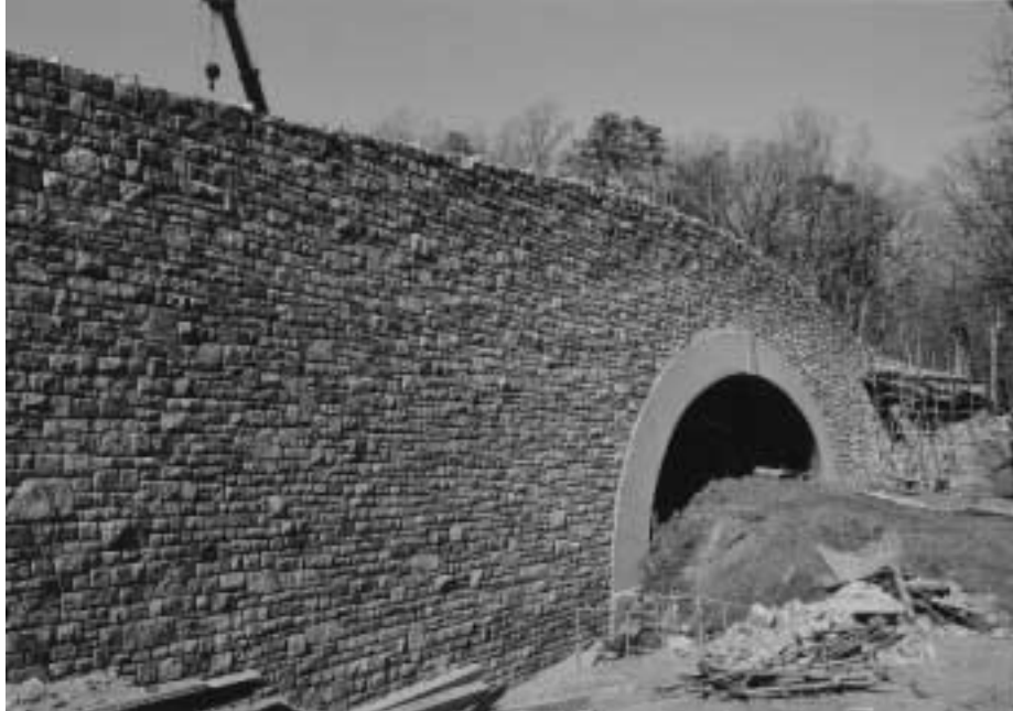
The eastern wall of Saunders Bridge, with fieldstone facing.
