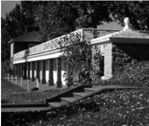
The South Dependency wing, which was completed in 1809, houses the Kitchen, Cook's Room, and other spaces.
